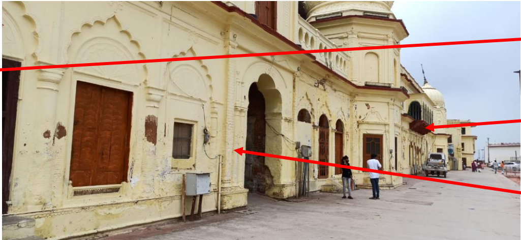
GANGA MAHAL: WINDOW, ARCH, PILASTER, PARAPET & CORNICE
