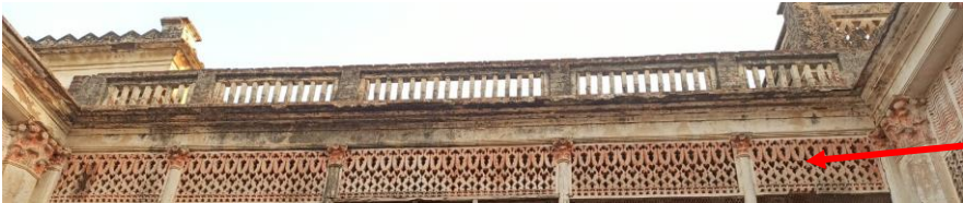
KANCHAN BHAVAN: PARAPET AND CORNICE
