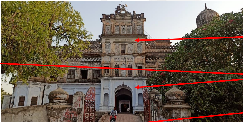
KANCHAN BHAVAN: WINDOW, ARCH, PILASTER, PARAPET & CORNICE
